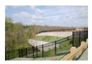
The Christ Hospital Green Township campus features a medical office building with both surface and underground parking, as well as space for a future expansion. Due to significant elevation change across the site, a series of retaining walls provide buildable pads for the buildings.
